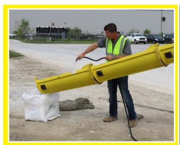
Wash water is any water that comes into contact with any material on a ready mix truck.
