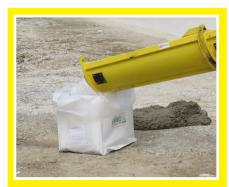
All ready mix drivers are responsible for determining if the washout container or pit is suitable to washout into.
