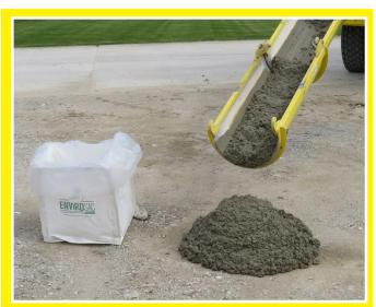
Left over concrete is not considered a pollutant and can be left on the jobsite as long as it does not come into contact with waters of the state before curing.
