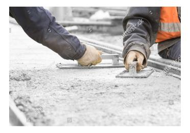
1. Do not place concrete on freezing subgrade.
